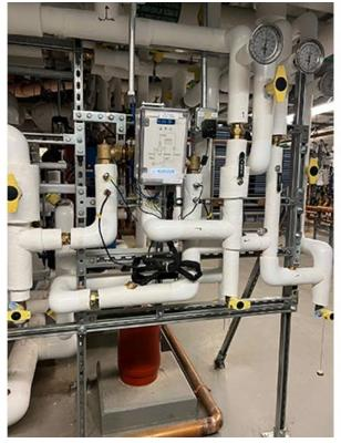
Leonard's Nucleus models give plumbing engineers complete system monitoring with outlet temperature control within +/- 2F from set point, regardless of demand. Features include user programmable set point, integral daily sweep and sanitization.
